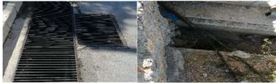
Figure 15: The Drainage System Separating the Rain Water from the Sewage on the Main (Kötekli) Campus
